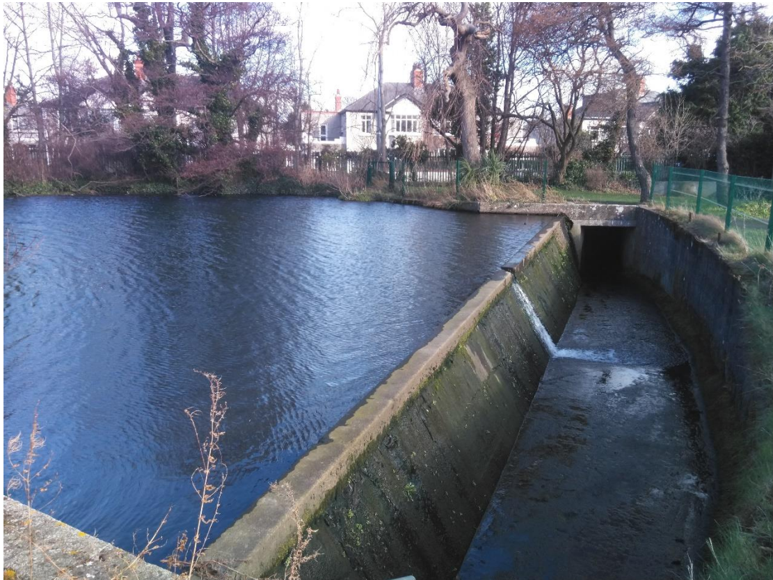
Image 1: Existing pond on site - Downstream Overspill and Discharge from site
