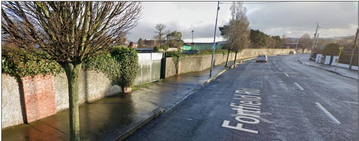
Figure 3-2: Existing Access on Fortfield Road (Photo from PUNCH site visit)
