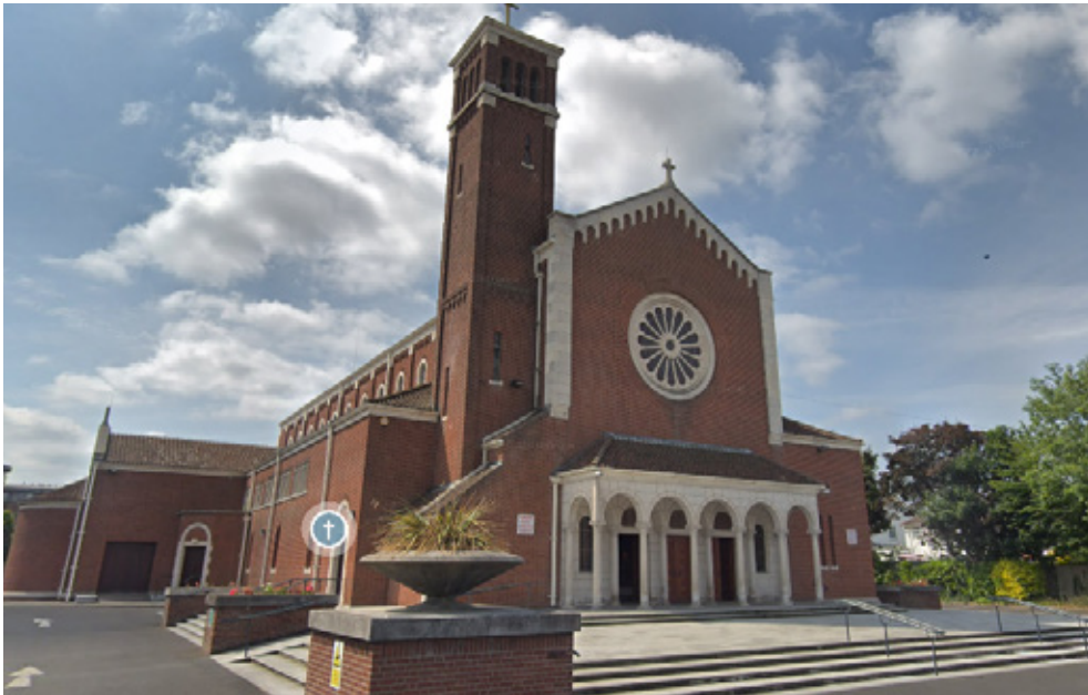
St Pius X-Roman Catholic Church with red brick facade and white granite highlighting architectural elements such as entrance, podium, cornices, parapet, window surrounds, etc.
