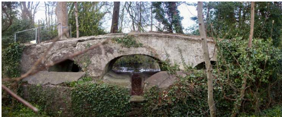
Figure 4.8 Brick-constructed footbridge and the eastern end of the lake. A small cascade under the central arch was the original outlet of the lake. The bridge sits on the dam which on this side is faced with a retaining wall. The haunching added to the arched openings is not original.
