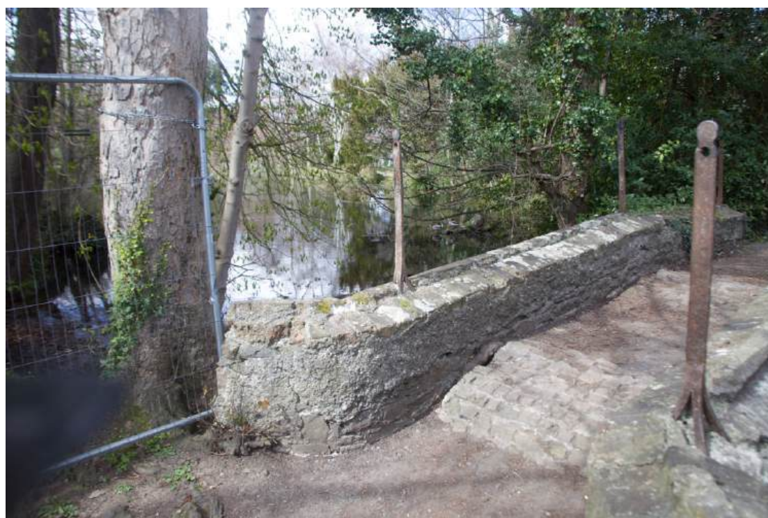
Figure 7.1 Stanchions crudely inserted in the bridge parapet
