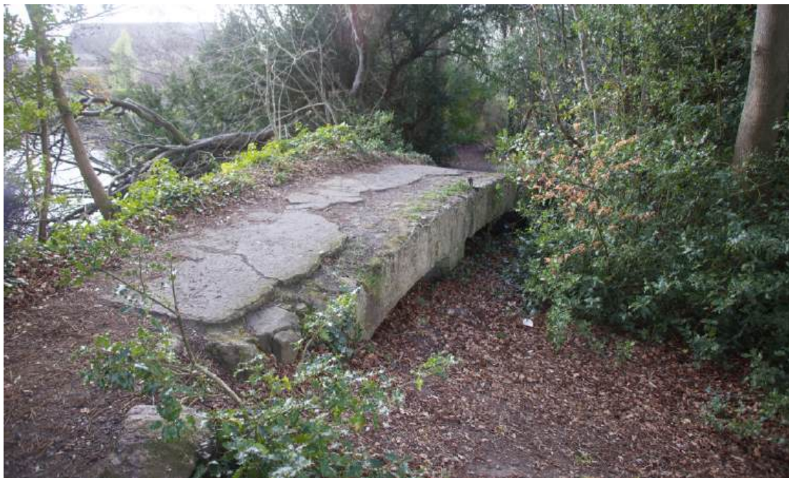
Figure 7.9 The single brick arch bridge. Currently it is propped at its centre by concrete blockwork
