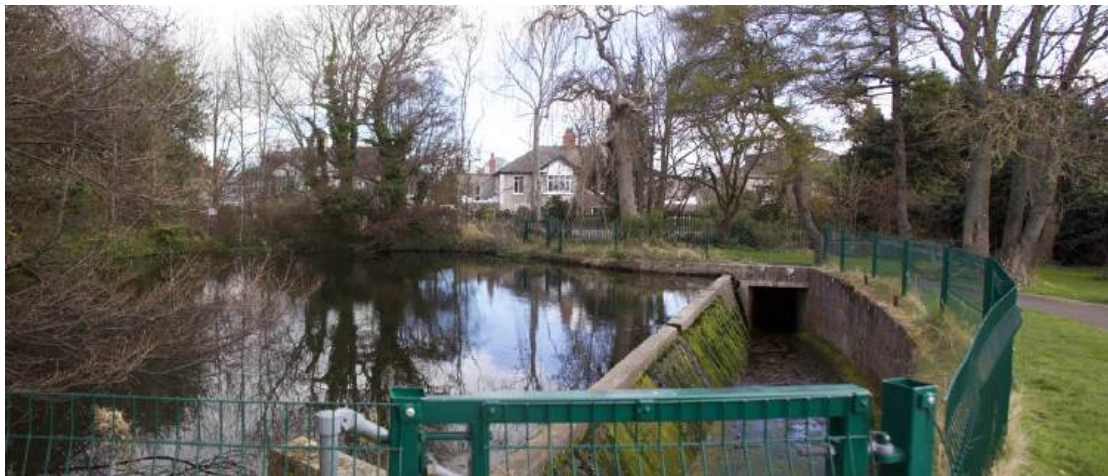
Figure 4.12 The current management of the lake's outflow constructed as part of the Poddle Flood Relief Scheme
