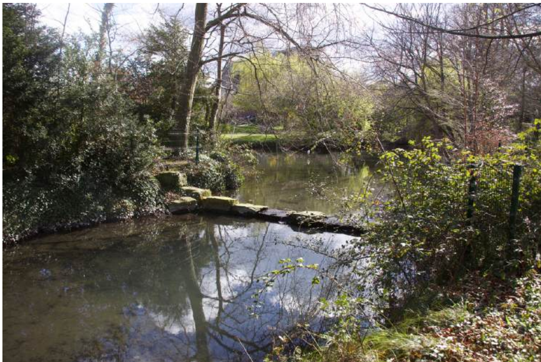
Figure 7.11 Miniature weirs on either side of the western island altering the water level at the eastern part of the lake
