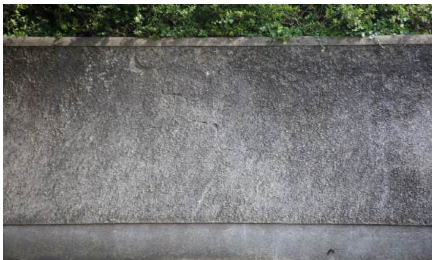
Figure 5 A section of the outside of the rebuilt demesne wall of concrete blockwork with cement render
