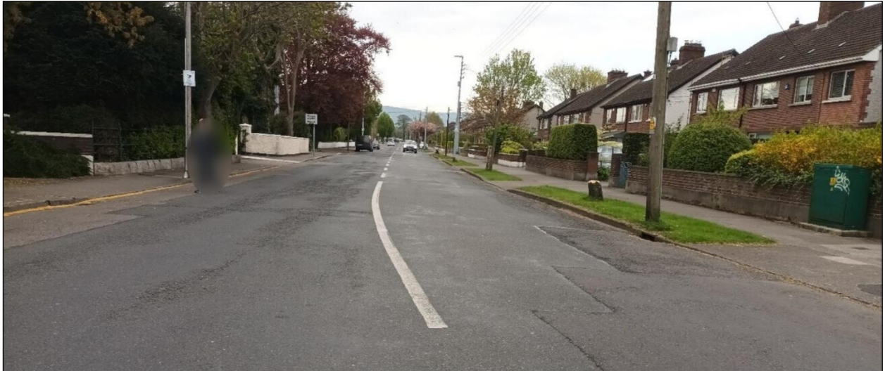
Figure 3-4: Fortfield Road (Looking South)
