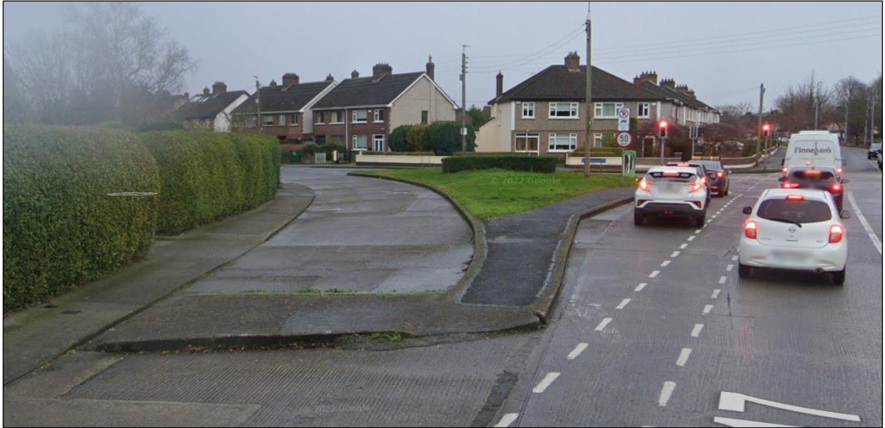
Figure 3-10: Now Closed Off Slip Road at Junction of Wainsfort Road and Fortfield Road (Looking South-West) © Google Maps
